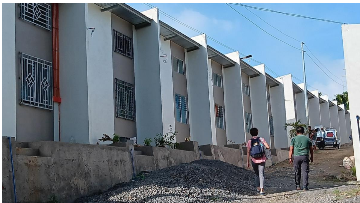
Figure 3. Retaining wall for the row of housing units
