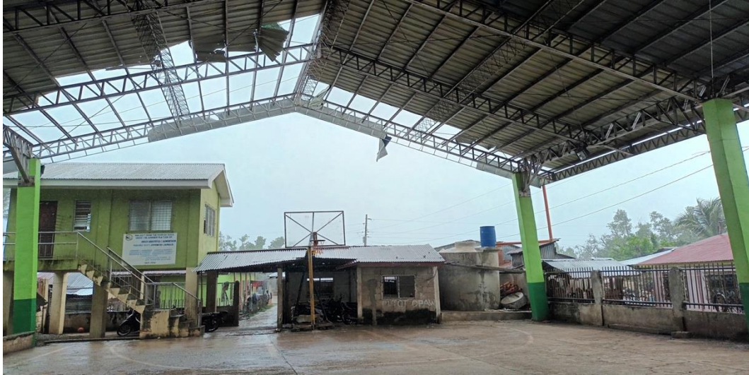
Figure 7: Rainwater catchment in partially damaged Covered Court of Barangay Cuya.
