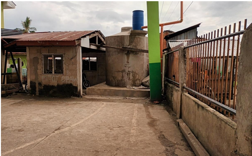
Figure 8: A closer shot of the rainwater catchment in the Covered Court of Barangay Cuya.
